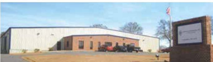
AIRCRAFT COMPONENTS AND GSE MRO FACILITY
